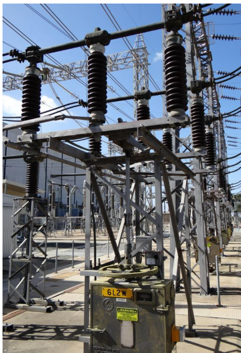
Figure 2 – 66 kV isolator at the Torrens Island A substation.
