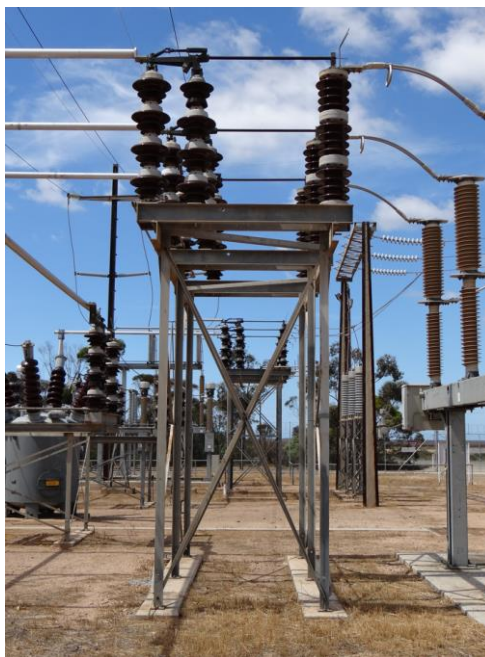
Figure 2 – 66 kV isolator at the Torrens Island A substation.
