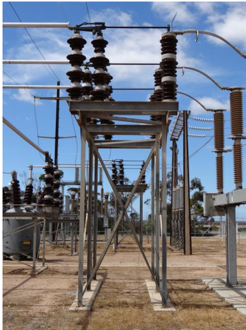
Figure 2 – 132 kV isolator at the Hummocks substation.
