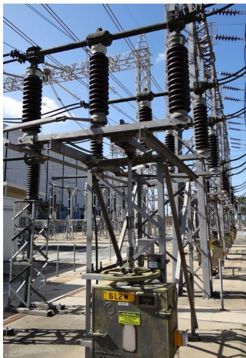
Figure 3 – 66 kV isolator at the Torrens Island A substation.
