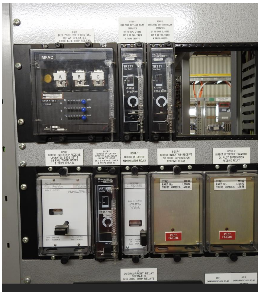
Figure 2 – Protection relays at the New Osborne substation identified for replacement.
