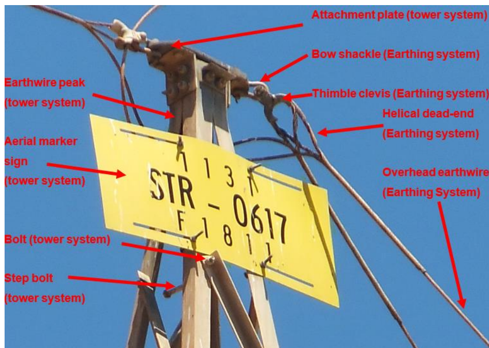
Figure 4: Structure system boundaries with aerial earthing systems
