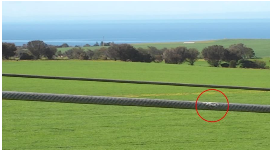
Figure 2 – Example of typical corrosion on the conductor and conductor hardware on F1803 Hummocks – Ardrossan West 132 kV transmission line identified for replacement.
