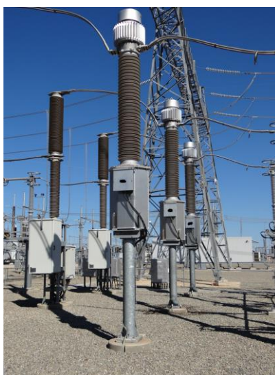
Figure 2 – Current transformers at Bungama substation.
